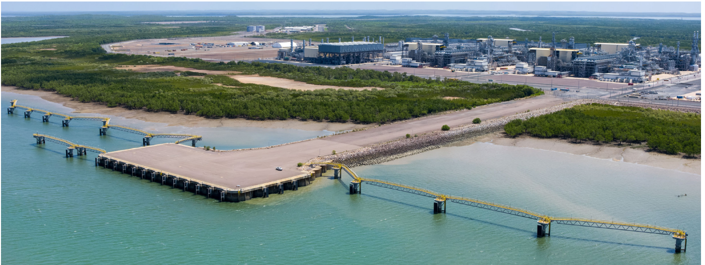
Figure 3 Berth pockets at the module offloading facility.
